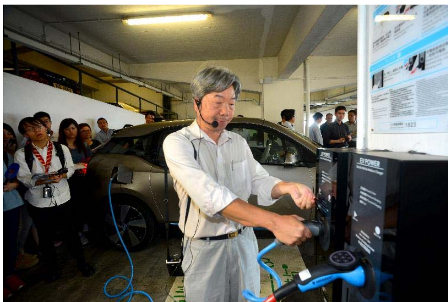
Staff from the Electrical and Mechanical Services Department explain how to operate EV medium chargers
