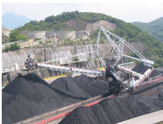
HK Electric Lamma Power Station Coal yard
