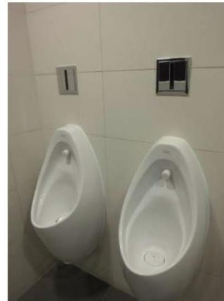
Sensor flushing for urinals
