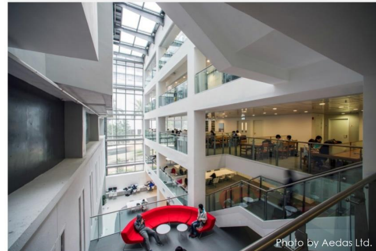
Skylights and Low-E glass walls between new and existing building
