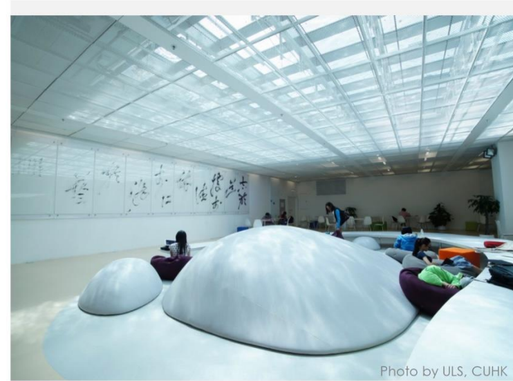
Under-pool skylights at LG/F with sun shading device, and the water also provides cooling effect to underground space
