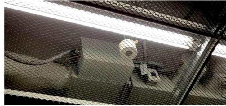
Adopted low flow low noise VAV A/C system
