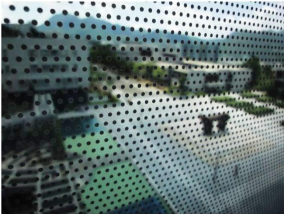
Low-E insulated glass panels with fritted dot pattern to reduce heat gain
