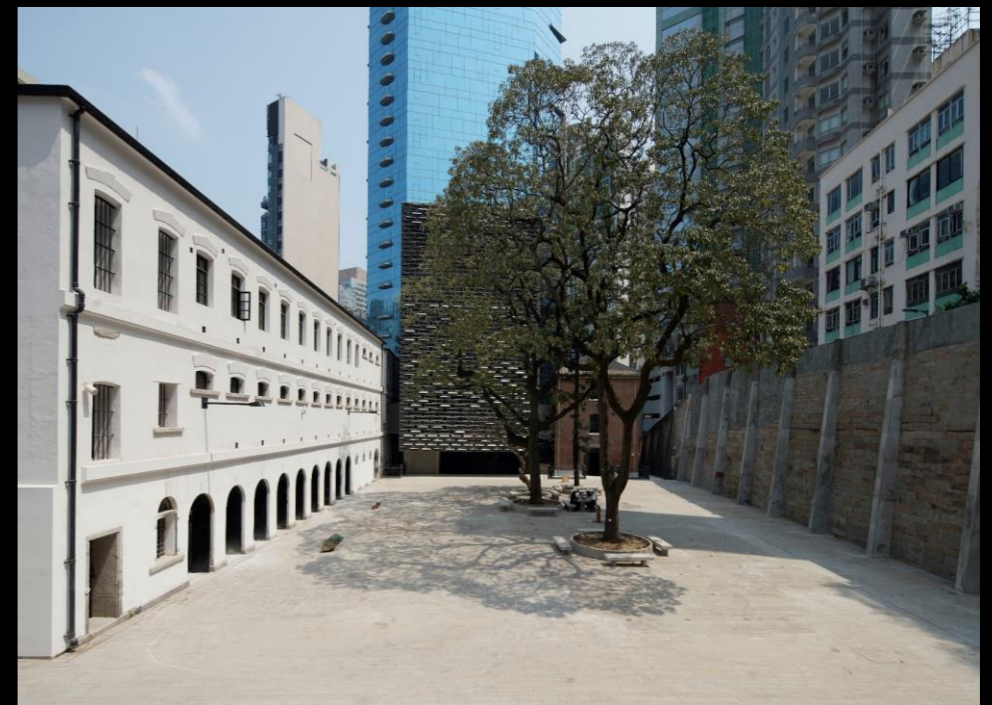
Underpinning strengthening work
