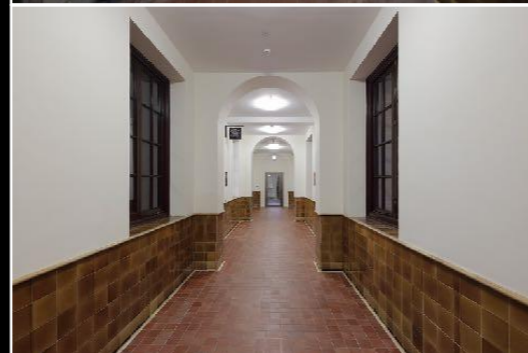
Floor and wall tiles
