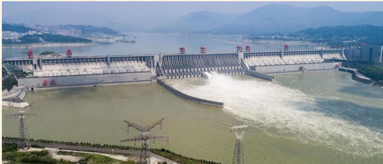
The Three Gorges Dam discharges floodwater
