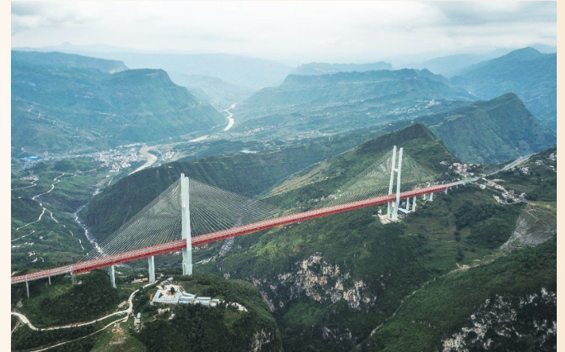
Beipanjiang First Bridge
