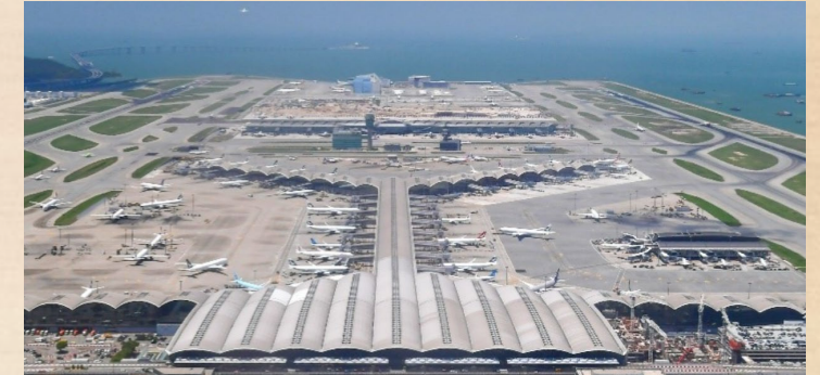
Hong Kong International Airport
