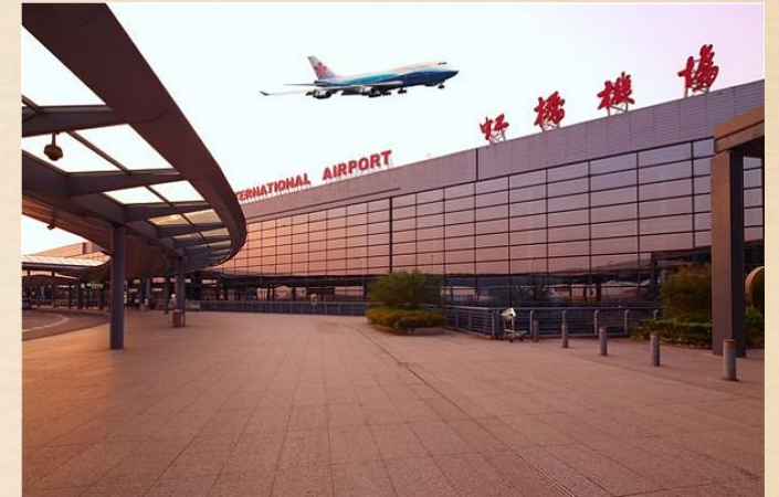
Shanghai Hongqiao International Airport
